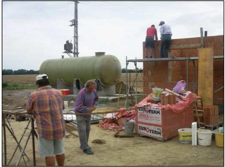
**Fig. 8. – Construction of pump house and the 20m<sup>3</sup> water tank made of fibreglass polyester**
