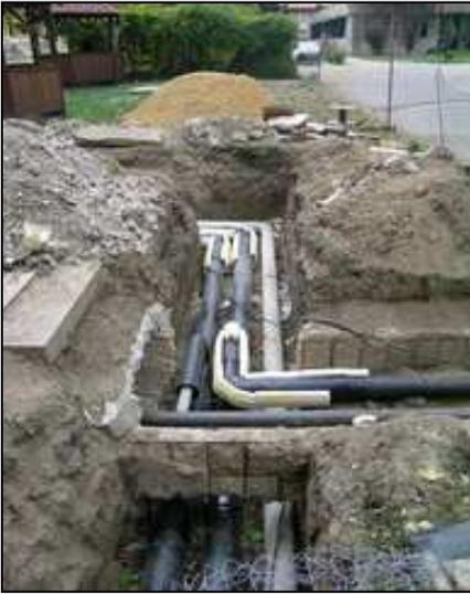
**Fig. 7. – Part of the three pipe system**
