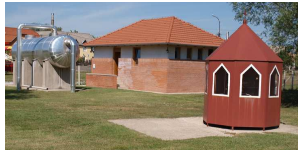
4. Figure Vicinity of well B-15
