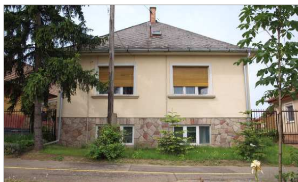
10. Figure Private house heated by geothermal
